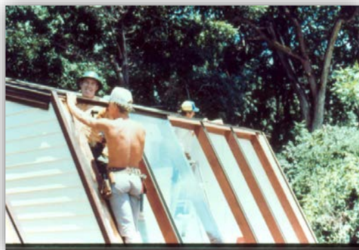
Figure 3. Hobby greenhouse being constructed with double glazed patio door glass.
